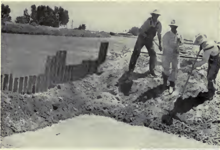
STOP GAP WALL made of sheet piling closes canal break. Note lightness of metal as Dave Remaly in the photo at right passes one to Pete Gillespie on the canal bank. Photo above, courtesy of the Twin Falls TIMES-NEWS; photo at right by Stan Rasmussen.
